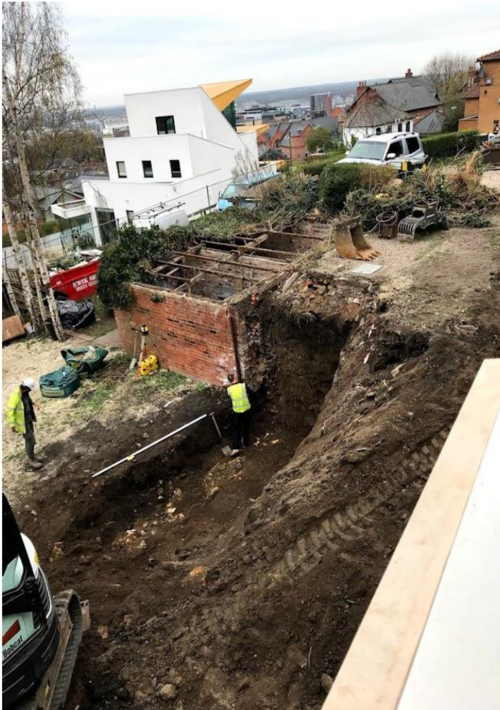
North-East aerial view of buttressing effect of outbuilding, also showing exposed wall top at circa 400mm, depth of wall estimated at 600-700mm at this point
