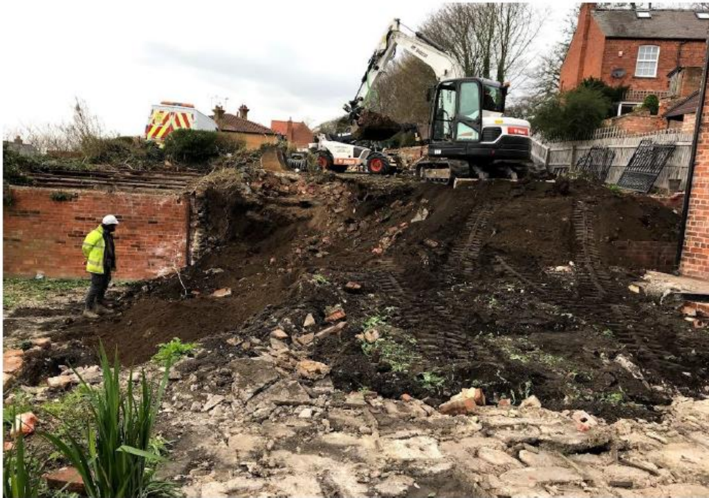
Wall failure at intersection with outbuildings
