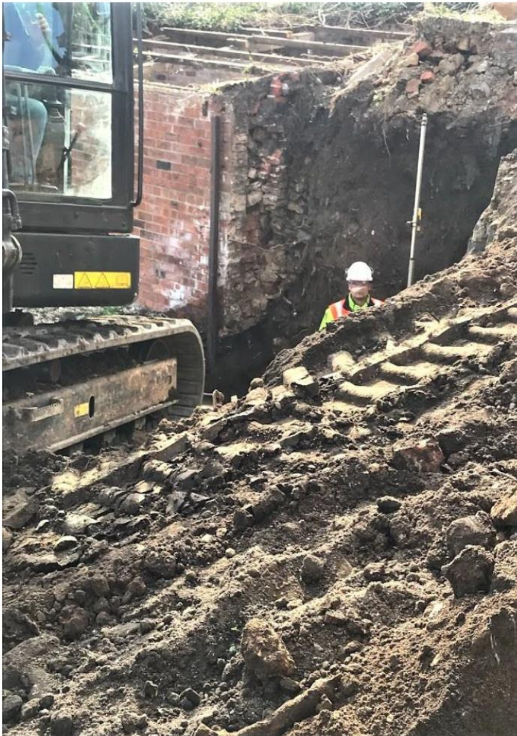
Alternative view of buttressing support structure of outbuildings – wall to wall abutment
