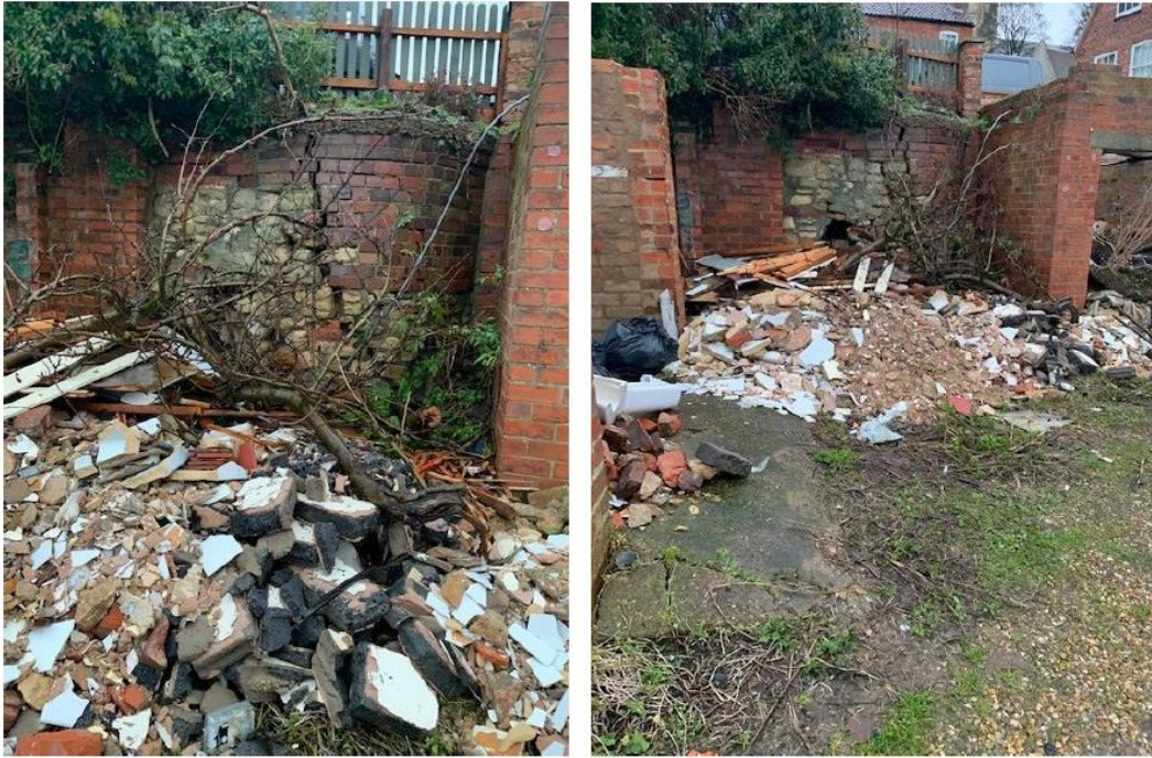
Images 1 & 2 - condition of existing wall
