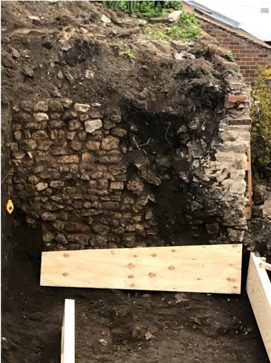
Northern retaining Stone wall cross section
