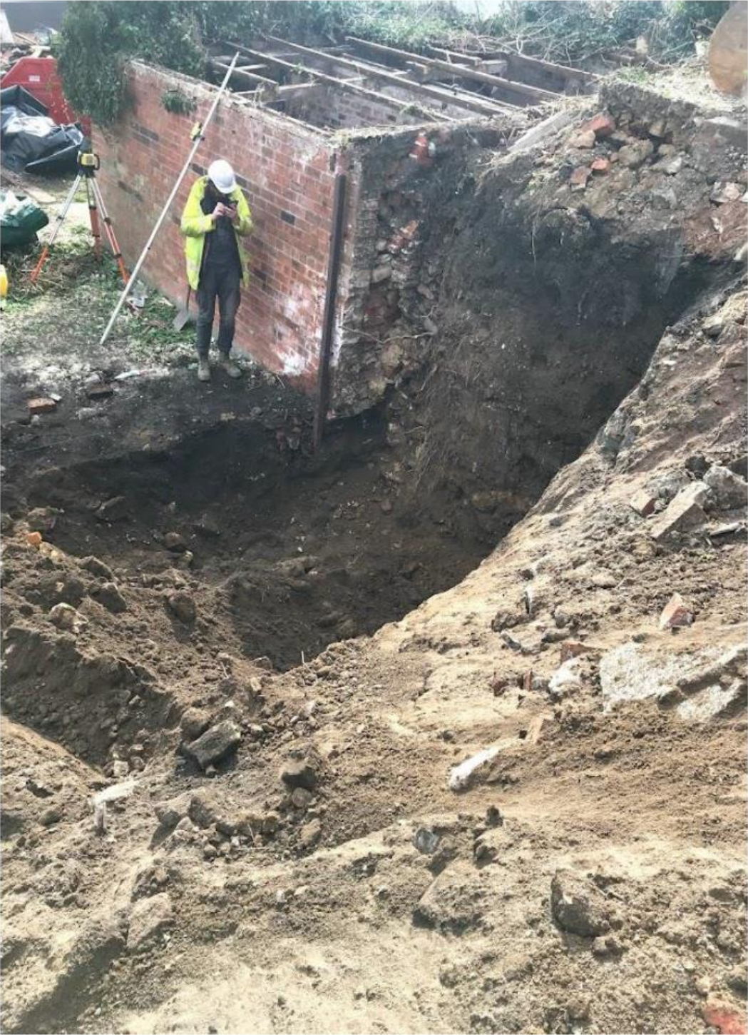
Viewing stone wall structure behind outbuildings and reliant upon the support
